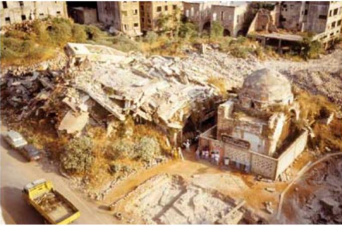
A heavily damaged Souks area in the city centre of Beirut ( https://www.world-archaeology.com/features/beirut-excavating-the-souks ).
