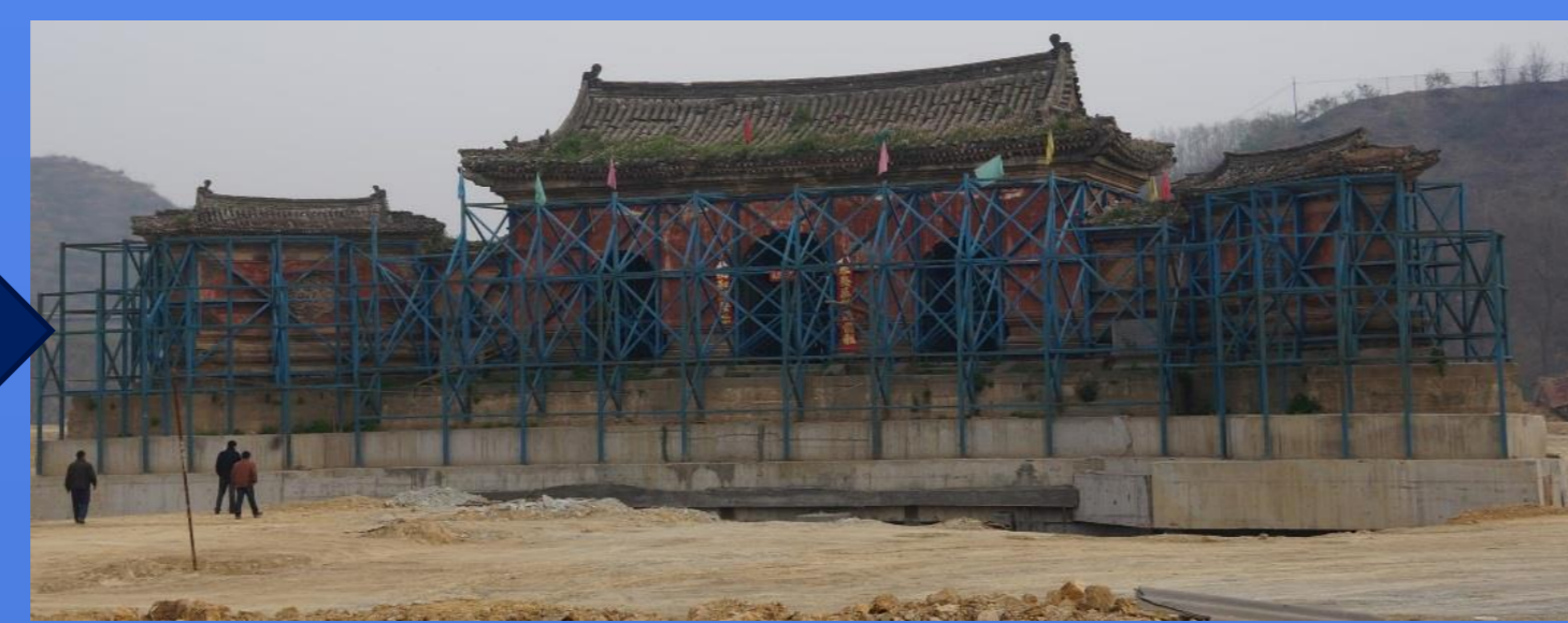
Gates after 15 meters in-situ elevation!
