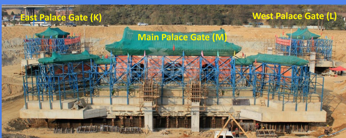
During the elevation: all the other buildings have already been dismantled
